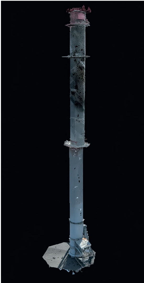
Fig. 2 | Central trunk (elevator shaft) extracted from the textured mesh of the Kyiv TV Tower and used to define the region of interest for verticality analysis
