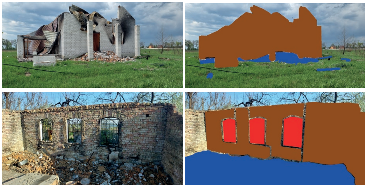
Fig. 1 | Examples of original (left) and annotated (right) images. Damaged walls are shown in brown, damaged windows in red, and debris in blue. Background and areas that are not damaged are shown with the original colours.
