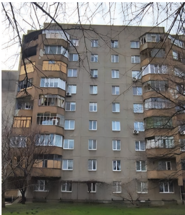
Fig. 2 | Part of the building's facades
