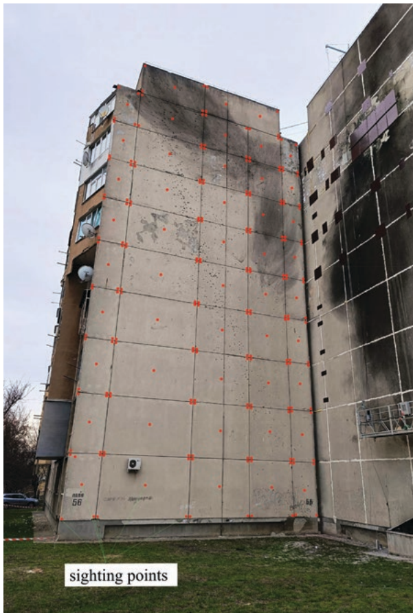
Fig. 7 | Scheme of the horizontal and vertical reference framework
