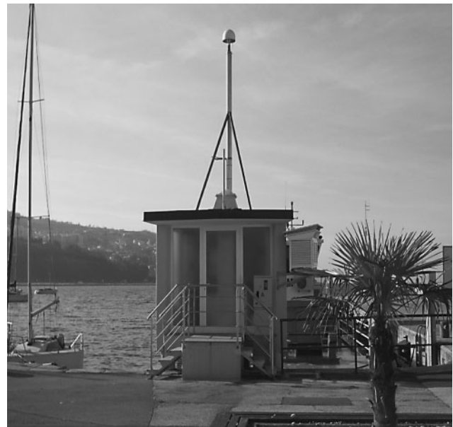
Fig. 3: Control point KOPE – GPS antenna or reflector
