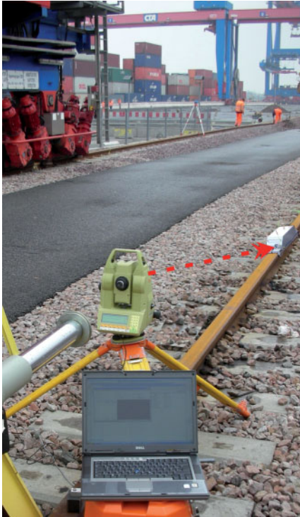
Figure 1: The Crane-Track-Surveying-System (CTSS) „Rail-Control“.
