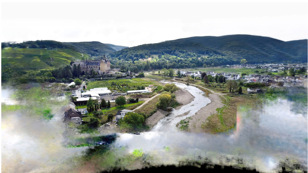
Fig. 1: Neural Radiance Fields NeRF model based on data extracted from a drone flight southwest of Ahrweiler, Germany (NeRF model: SCHOB 2022; Drone imagery: REKITTKE 2022)
