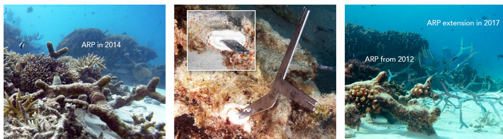
Fig. 5: Artificial Reef Prototype (ARP) in 2014 (left) and its extension (right) in 2017 in Gili Trawangan, Indonesia. The removed CaCO 3 layer of the five-year-old structure exposed a fully functional push-to-fit connection to connect new construction elements with an existing structure.
