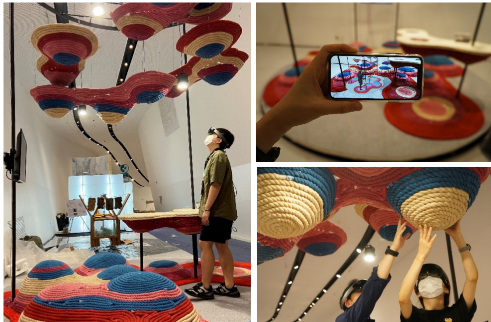
Fig. 6: On-site installation supported by HoloLens and exhibition with web AR model
