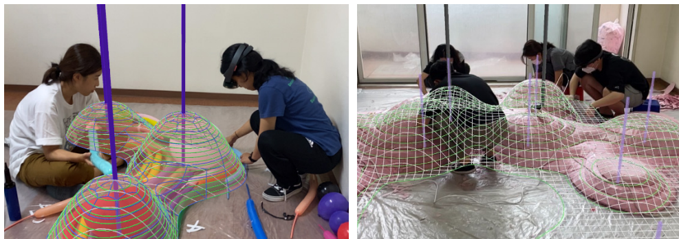
Fig. 2: Shaping with balloons and cutting Styrofoam (view with AR holographic model)
