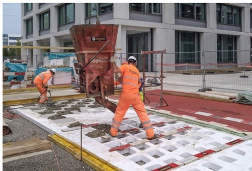
Fig. 6: Mold prototypes cut from polystyrene with a water-jet cutter (CNC-controlled) (Source: WEINSBERG (2018, May 13), personal communication May 13, 2018, Image © BRYUM)
