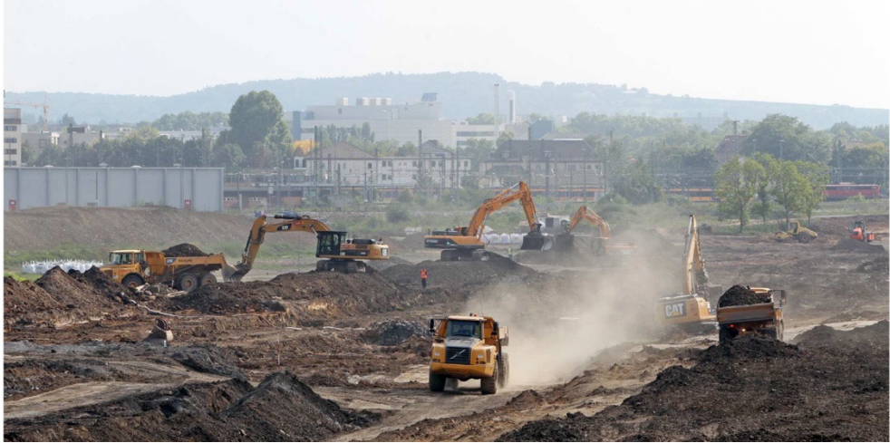
Fig. 1: Excavations at the Summer Island
