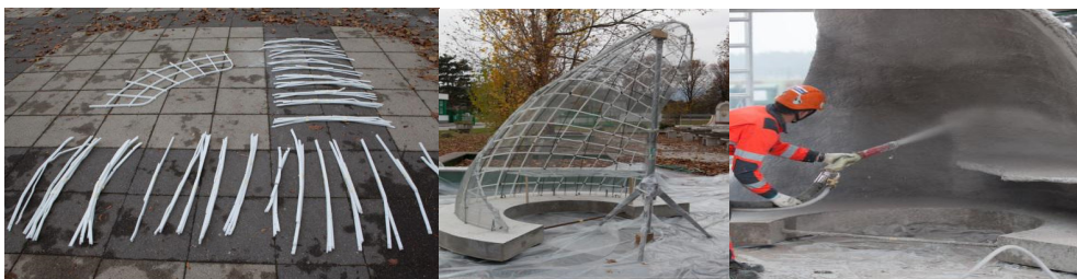
Fig. 3: On site installation of Clever Contour technology (© Clever Contour GmbH)
